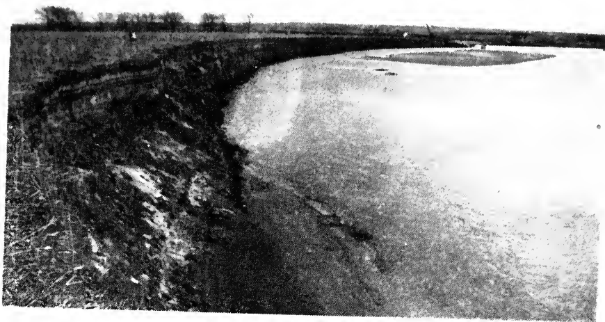
Fig. 1—Severely eroded river bank.
